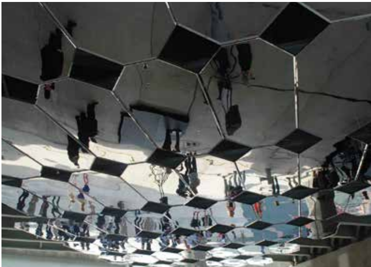
Reflective ceiling installation example
