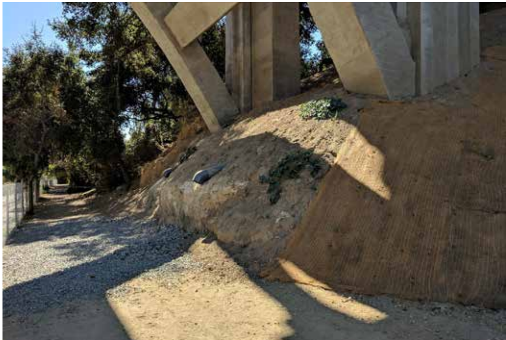
Trail Erosion / Surface Water Run-on
